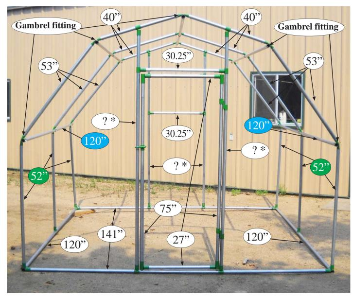
1) Assemble base first, using your 4 corner fittings. Be sure to slide on your "T" fittings before attaching tubing to corners. Insert the self-tapping screws into the corner fittings.
